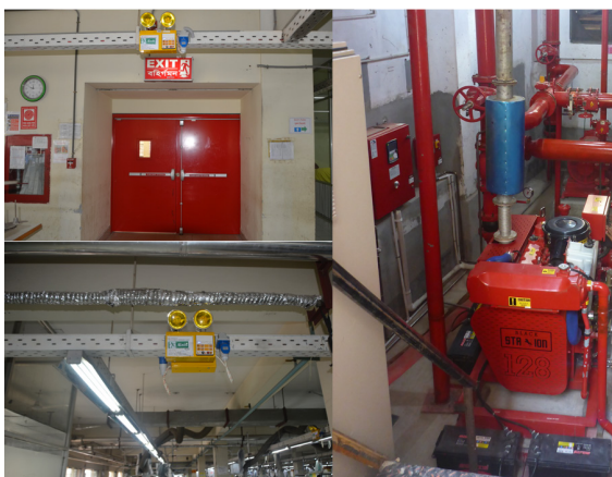
Example of fire safety remediation at Accord-covered factories.
